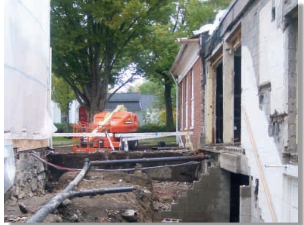
Two stages of the separation of the Baldwin House from the former library building by Welty Building Company, Ltd. workers.
