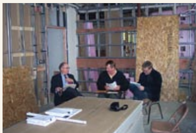
John V. Frank discusses restoration plans for the Baldwin House with contractors.
